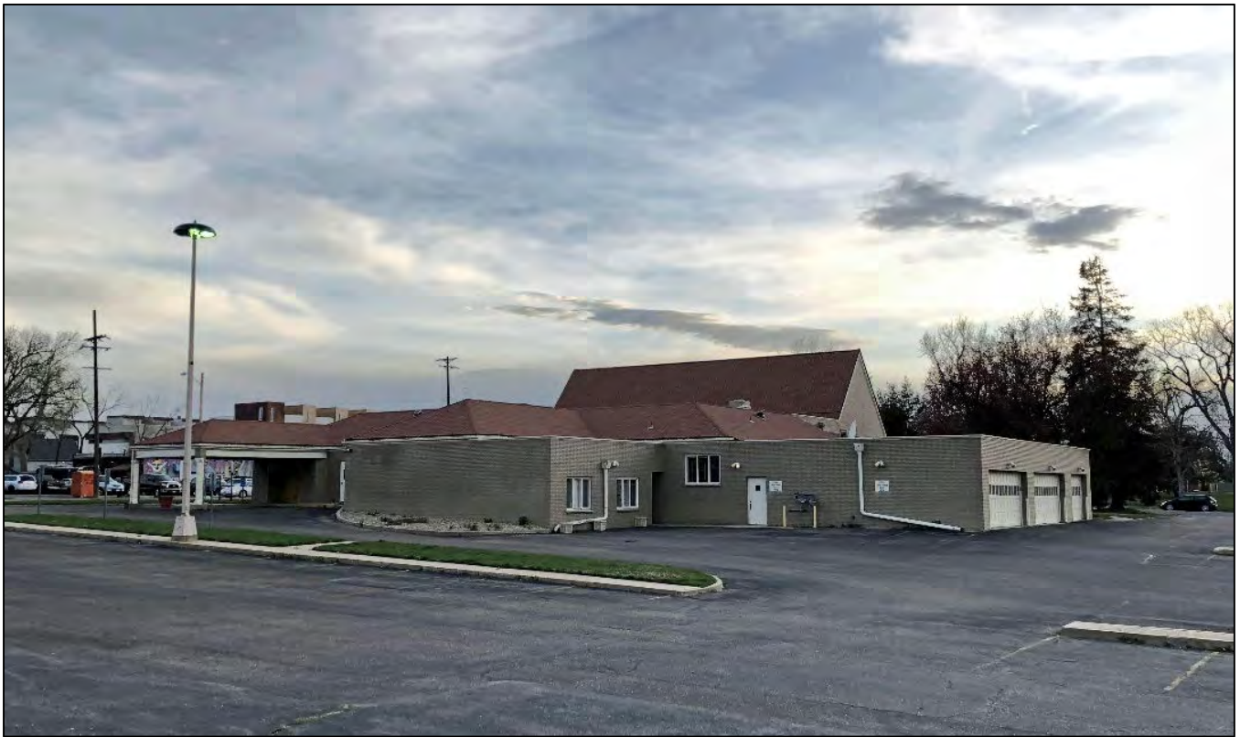
14. East wall and rear. View west-southwest, April 2018.
