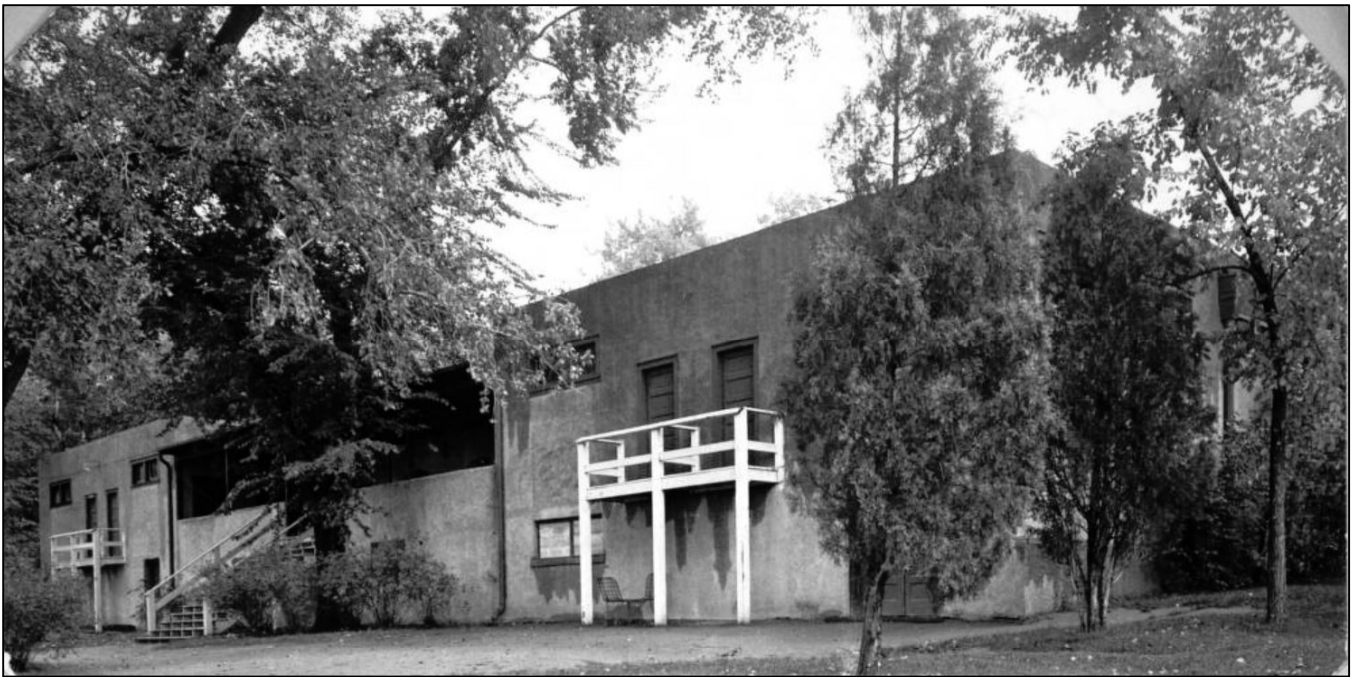
Rear (north) and west wall of bathhouse (view southeast). SOURCE: image number X-20283, ca. 1930-50, Western History and Genealogy Department, Denver Public Library.
