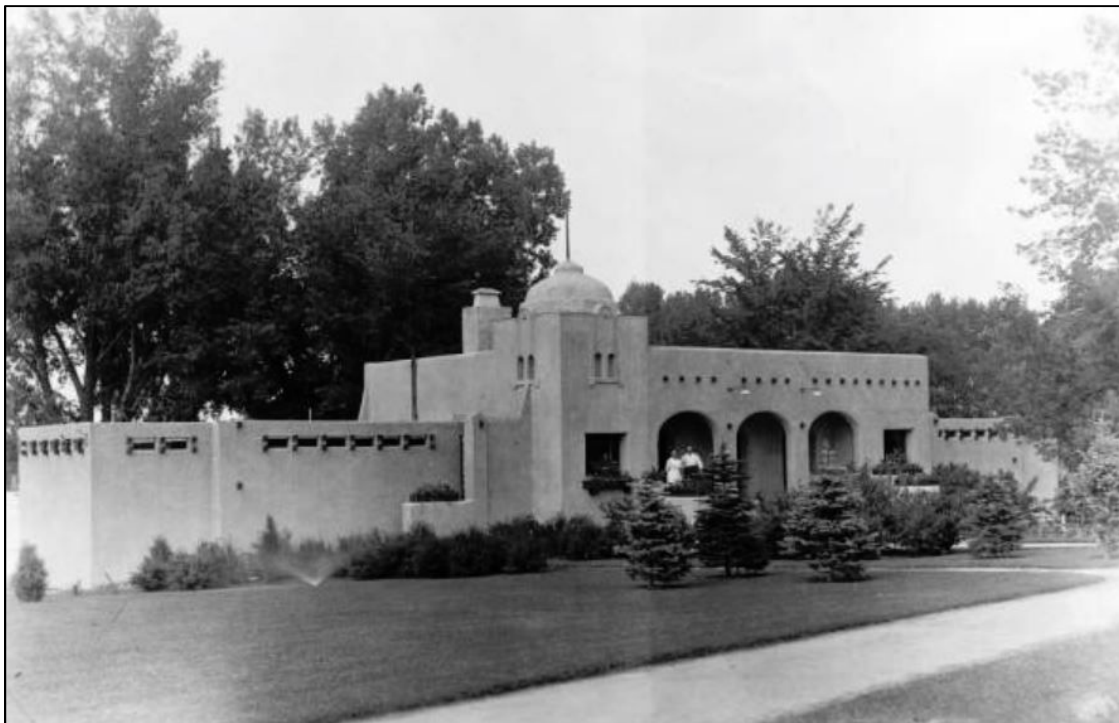
Front (south) and west wall of bathhouse (view northeast). SOURCE: image number X-27148, ca. 1918, Western History and Genealogy Department, Denver Public Library.
